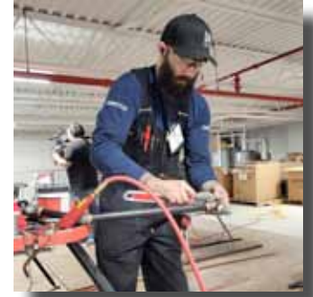
Apprentice Plumber Dave Young
